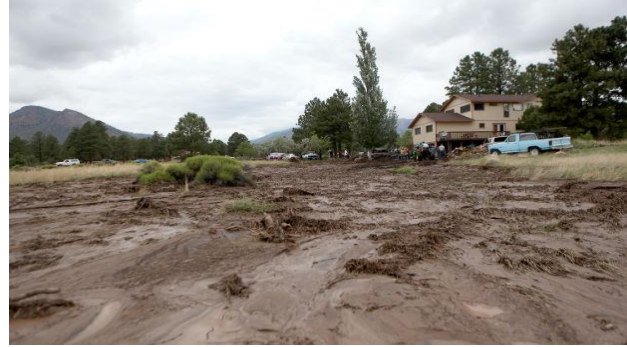
Significant post-fire flooding from the Schultz Fire near Flagstaff, AZ, required immediate mitigation of hillsides, roads, and slopes. (Photo: J. Bacon)
