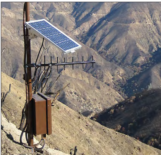
Original rainfall and telemetry station established after the 2009 Station fire in California. Photograph by U.S. Geological Survey.
