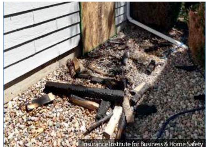
Figure 12: Embers ignited a firewood pile located next to the garage of this home. The direct flame contact exposure from the burning firewood ignited the composite wood (hardboard) siding product. Source: IBHS.
