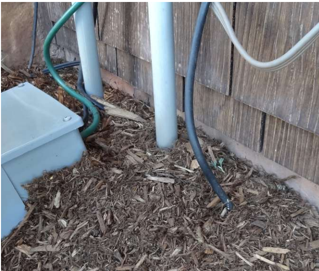
Figure D6: The upper photograph depicts the vegetation management (defensible space) in the 0-to-5 foot zone on the right side of the house. The lower photograph shows low earth-to-siding clearance. Source: IBHS.
